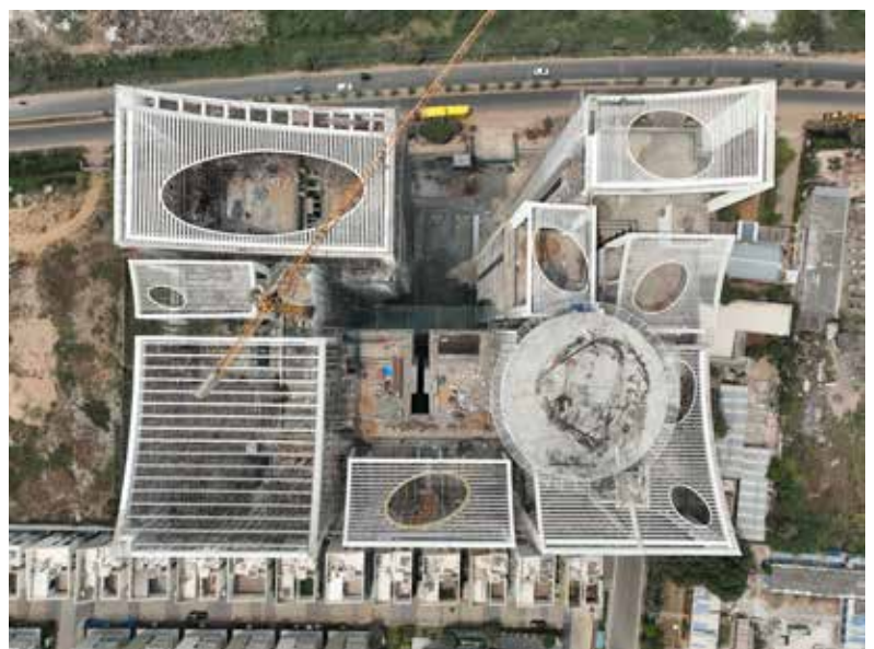
Current Site progress
